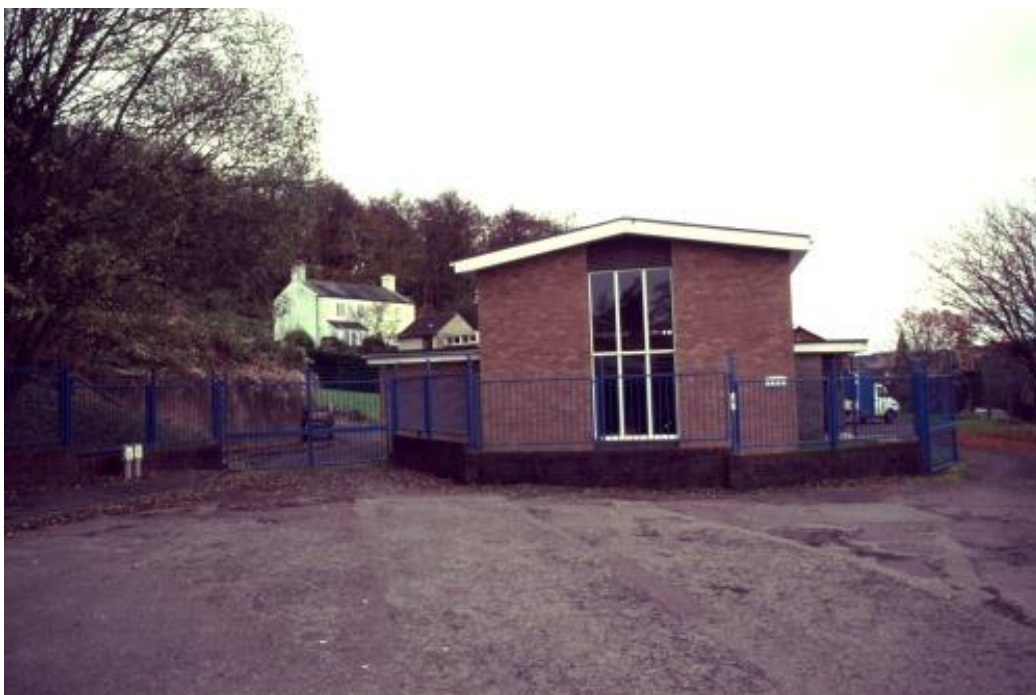
Pumping station above Buckshaft mineshaft (SO 654 121) looking south
