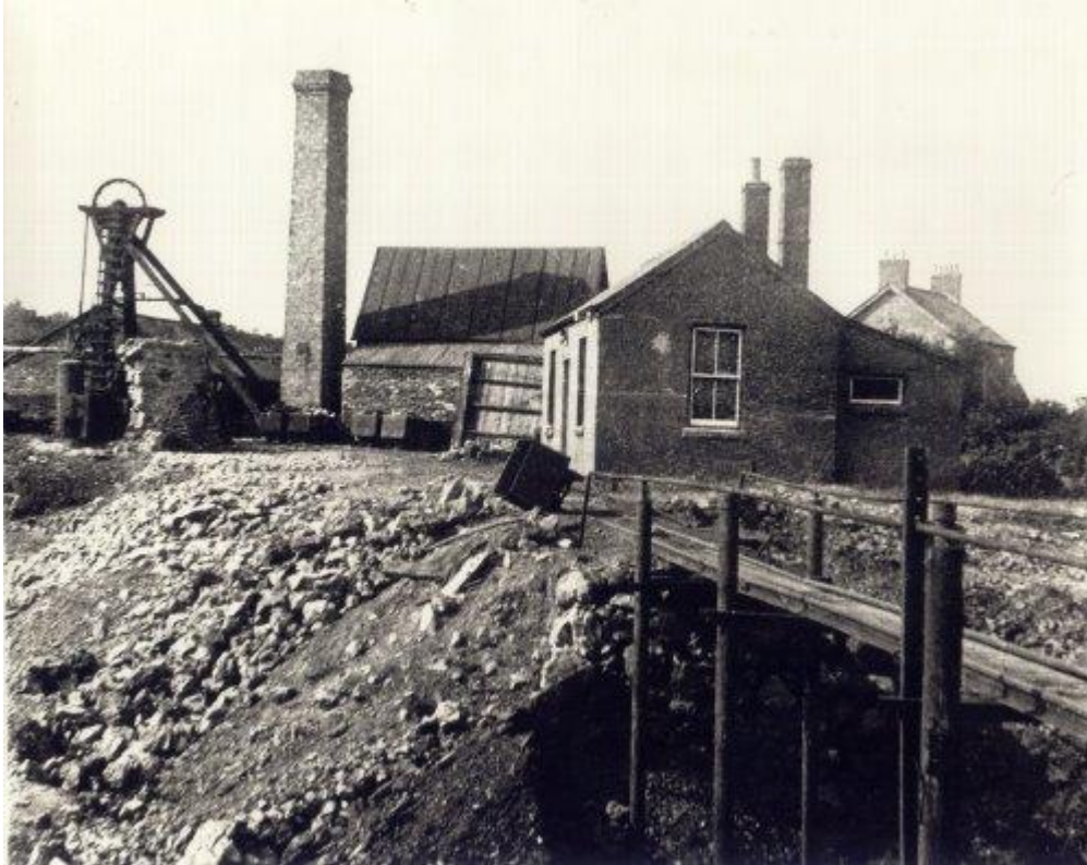
New Dunn Iron Mine
