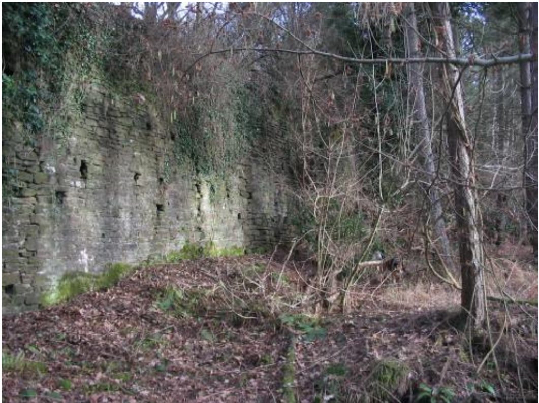
A wall near the shaft
