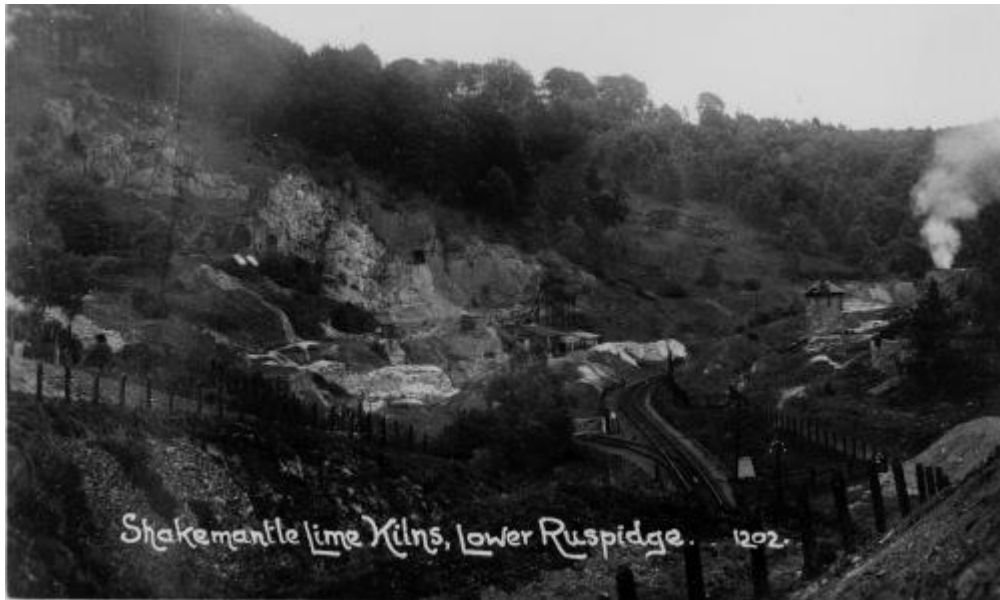
Perseverance engine house is on the right of this photograph
