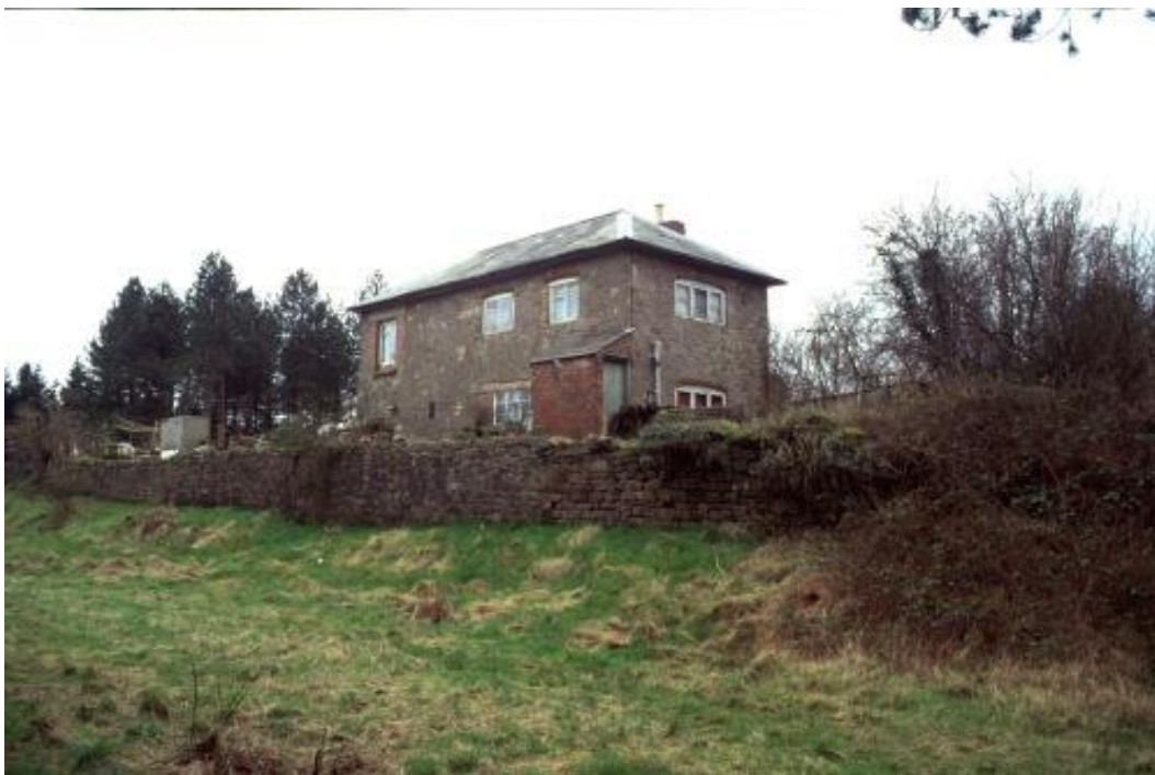
The former engine house (SO 652 194) looking SW
