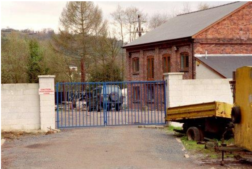
Converted buildings on the mine site
