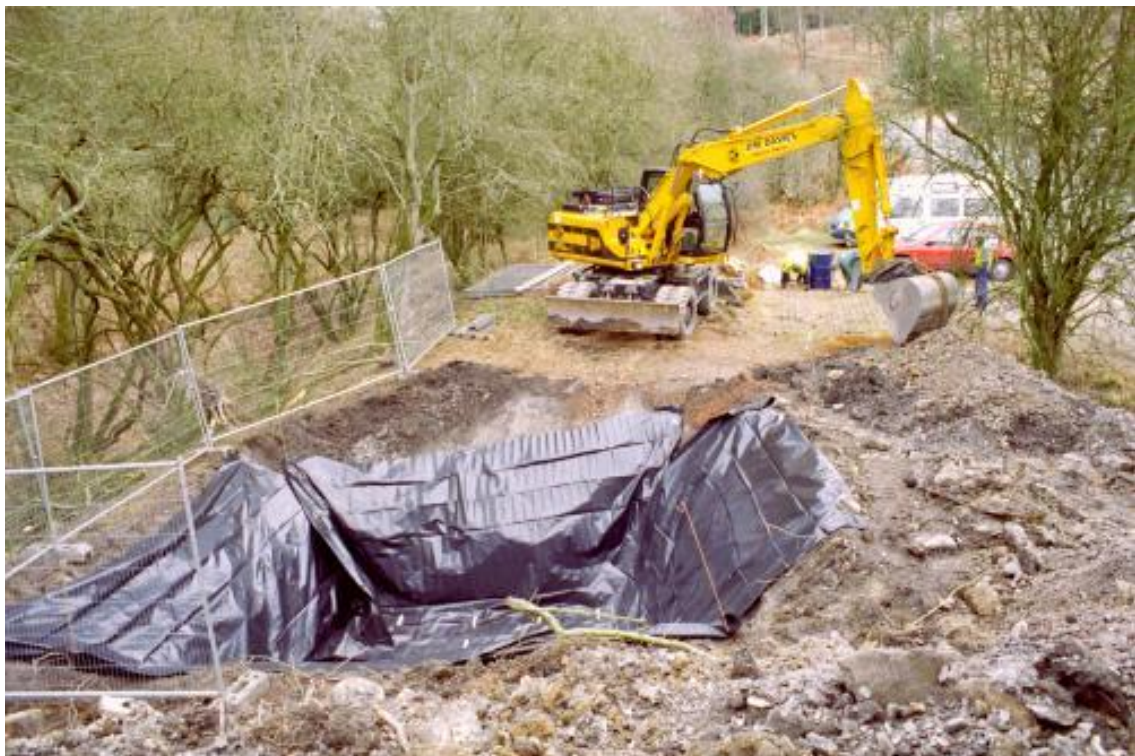
Digging out and infilling main shaft
