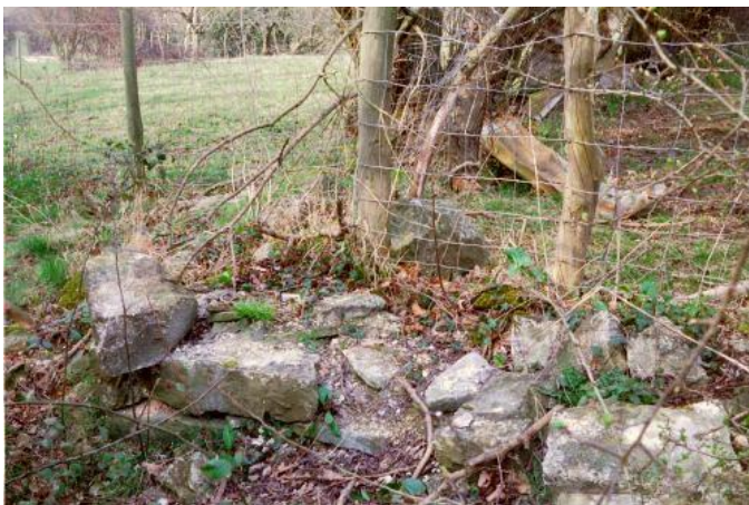
Masonry at Moorwood, looking N
