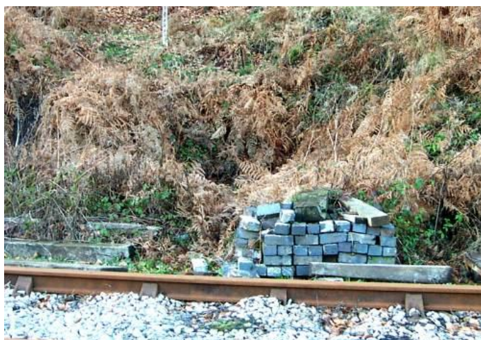
Site of Norchard level, looking south
