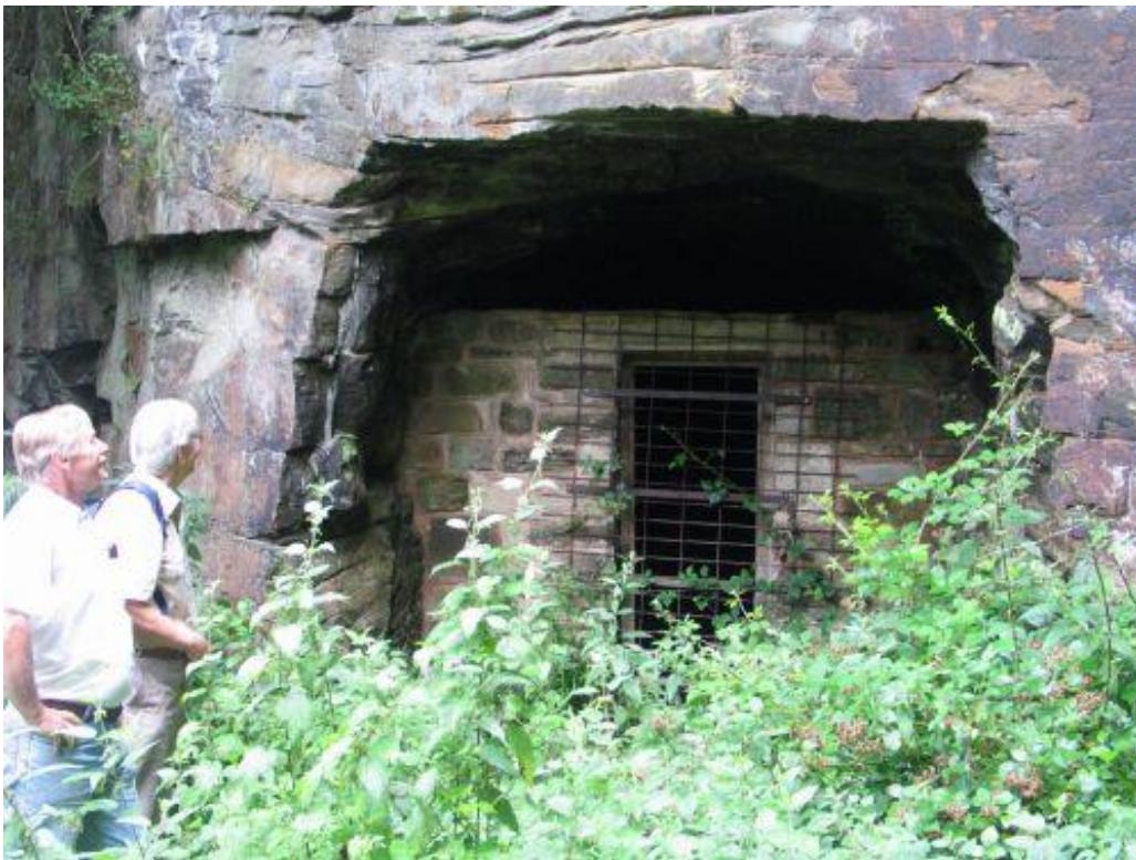
Trafalgar to Strip- and-at-it tramway tunnel entrance (2) (SO 62424 14468) looking NNW
