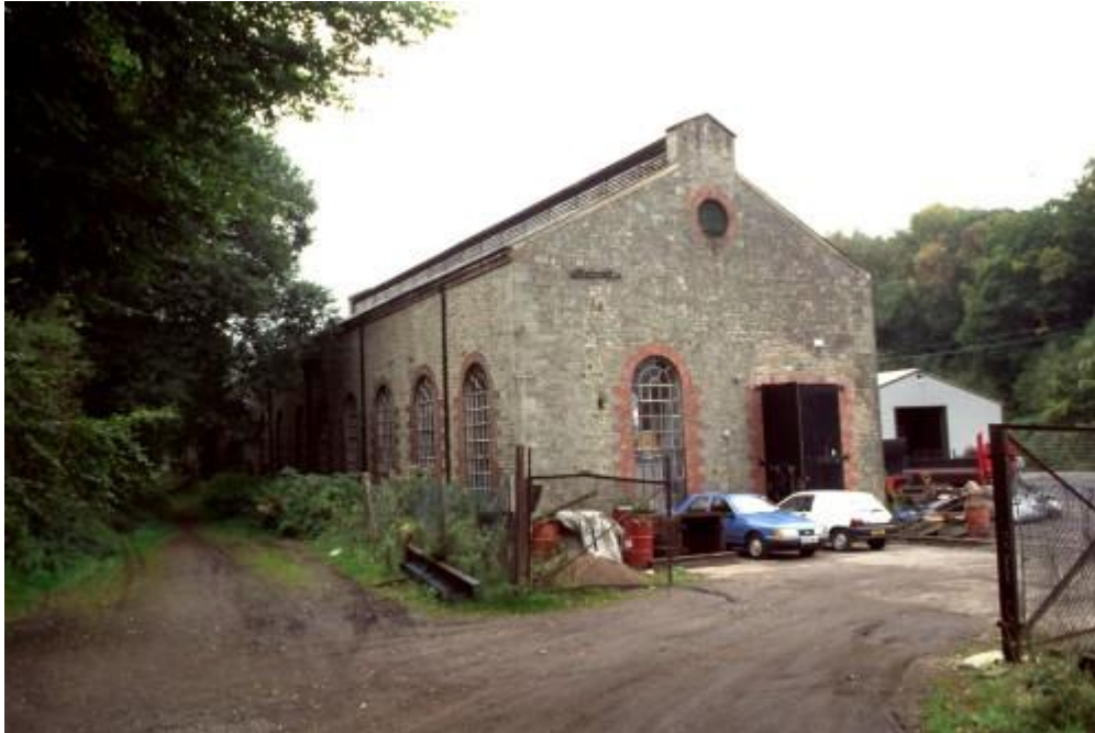
Flour Mill engine house (SO 6046 0679) looking SSW
