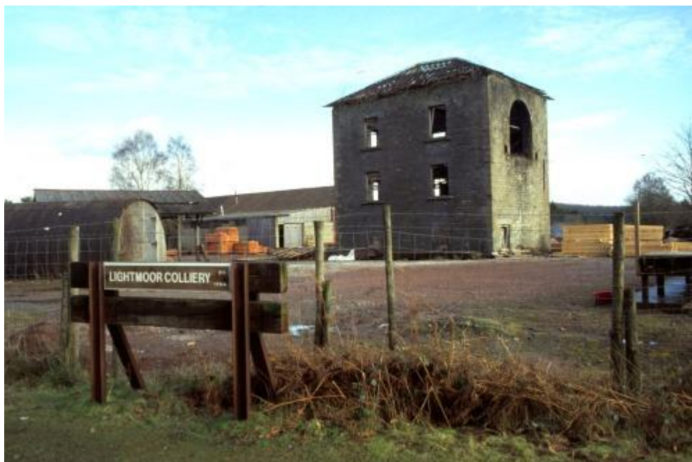
The former engine house (SO 642 121) looking SE
