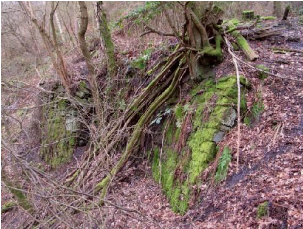
Stonework remains, looking SSE
