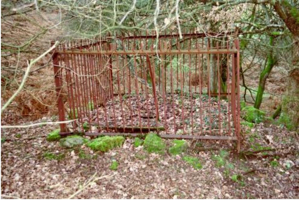
A capped airshaft on Tufts Level (SO 61903 04848) looking WNW
