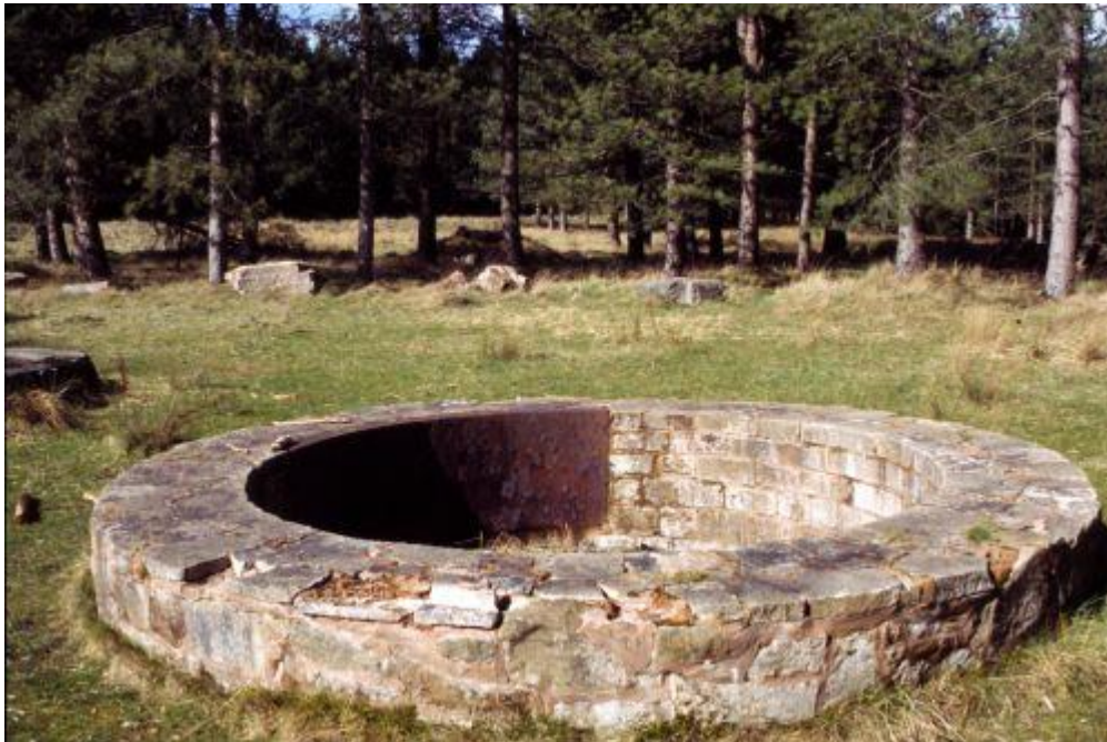
Site of New Bowson Shaft (SO 6438 1510) looking NW
