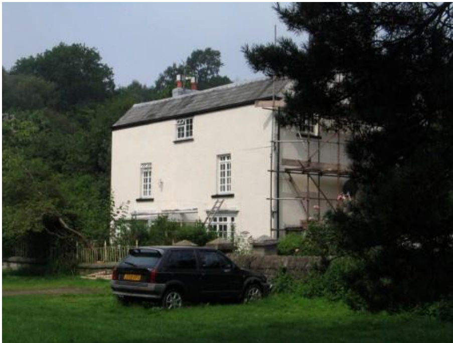
Trafalgar House (1), (SO 62579 14443) looking WNW
