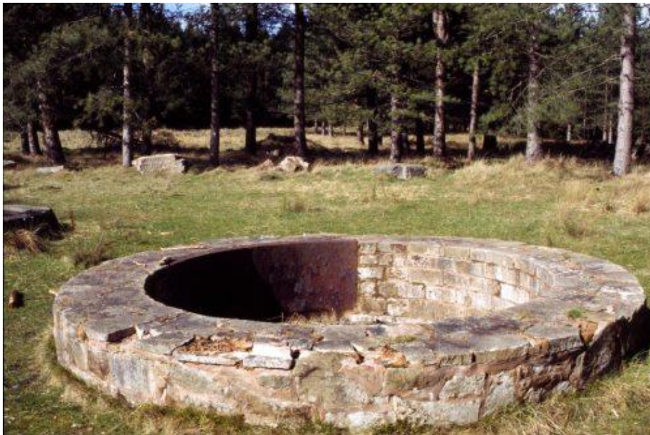
New Bowson shaft, looking NW
