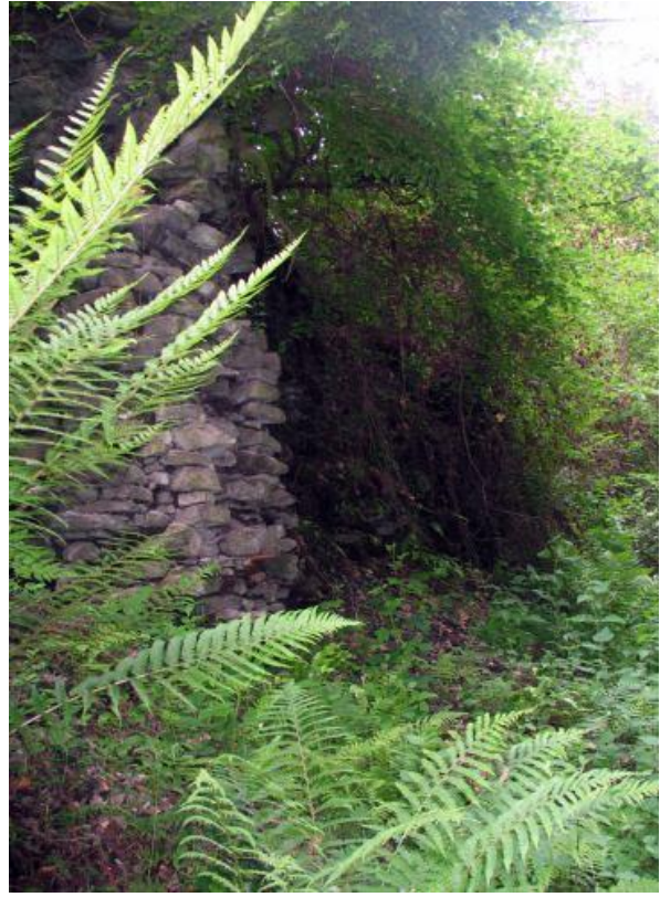
Stone bridge abutments, looking SW
